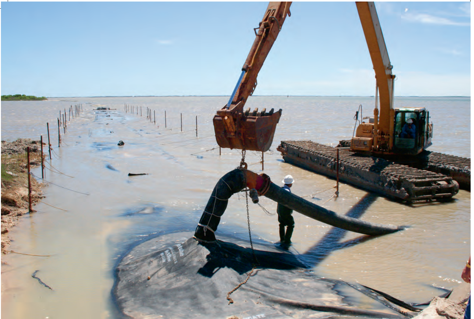
GEOTUBE® container being filled with dredged material.
